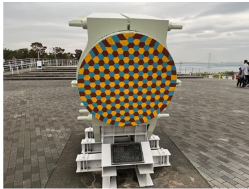
Awaji Suspension bridge; Karl in front of the bridge; an actual sized model of how the suspension cables are constructed.
